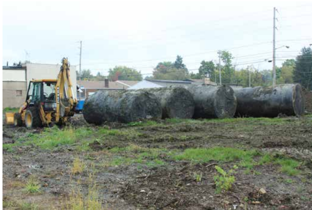
Underground storage tanks were removed at the construction site of the Glenwood Community Park. The presence of USTs can significantly delay a project and add to its cost.
