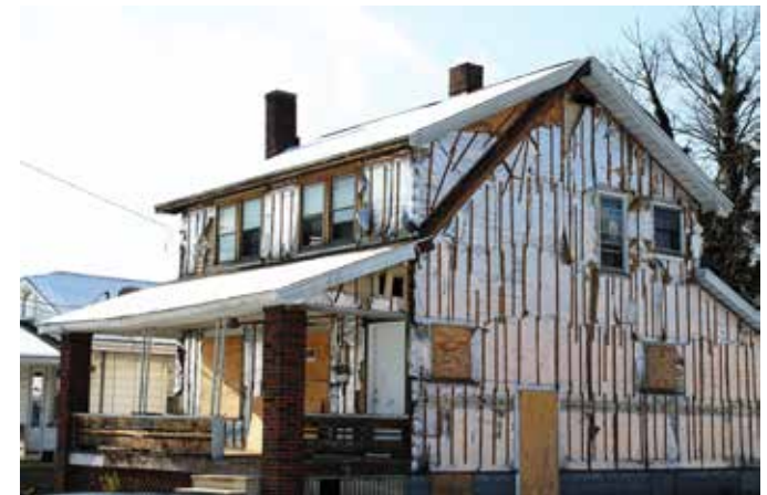
Major housing and property issues identified by residents included vacancy and blight, as well as dumping of trash and debris.
